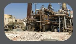
4-Electro-Mechanical Construction works for Conversion project for Boilers No. 1& 2 to work in natural gas instead of heavy fuel oil, including installation fan, ducts, steel structure and insulation works, with Arab Potash Co. (APC).
